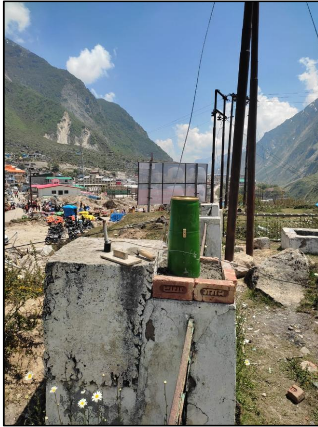
Figure 12: Rain gauge installed at the PWD office in Badrinath
